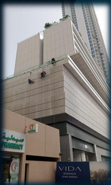
Client: EMAAR DEVELOPMENT P.J.S.C. Project Name: VIDA Residence, Dubai Marina Scope of Work: External ACP Façade & Glass Cleaning
