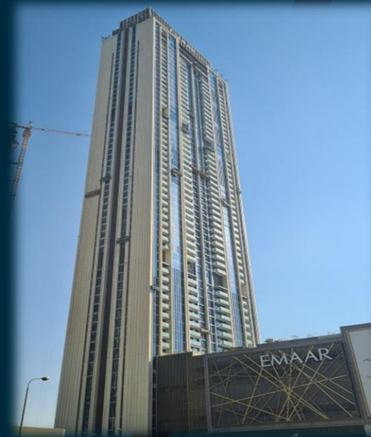
DOWNTOWN VIEWS RESIDENTIAL TOWER
